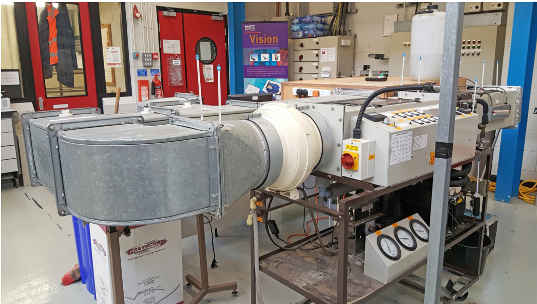
Institute of Technology Tallaght - features customer fitted recirculating duct
